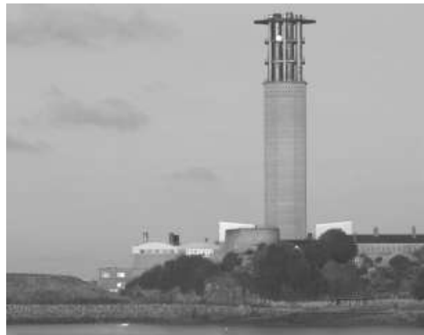
La Collette Power Station, Jersey
