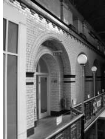
Haven Road Interior showing the ceramic tiles and balustrade
